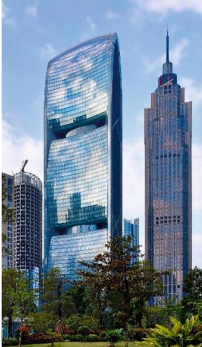
Pearl River Tower, Guangzhou
